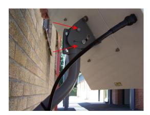
Figure 4-14 - Adjusting elevation
